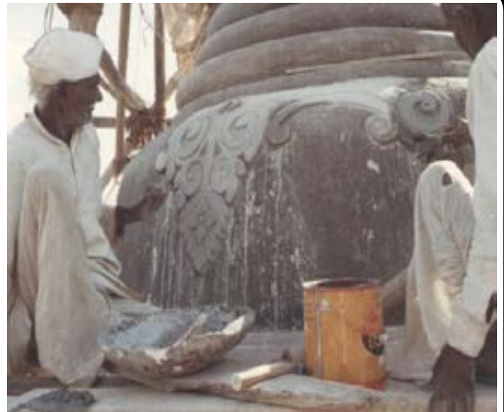
Masons working on Pagoda roof (early 1979)
