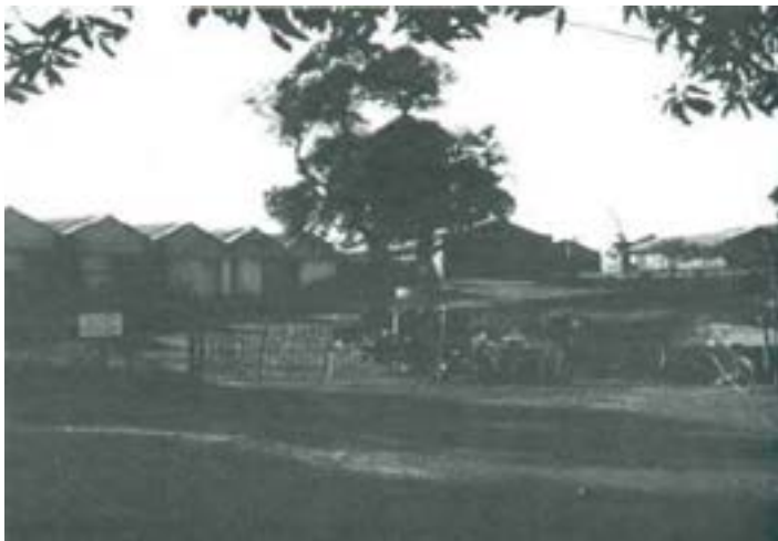
Entrance to meditation compound; beyond, new construction (1975-1976)
